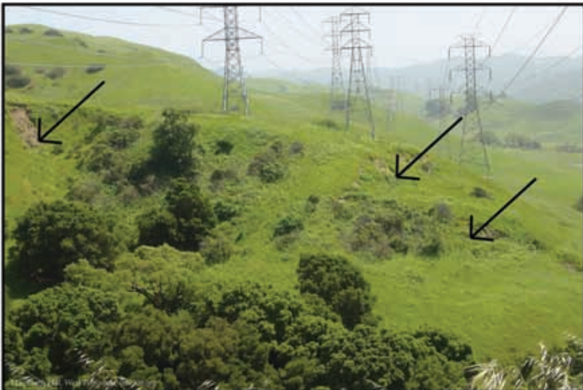
Photo 32: Slumping Soils at West Edge of Project (April 2006)
