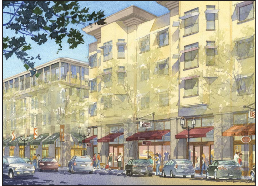
Artist Rendering of Sycamore North Development which is currently under construction
