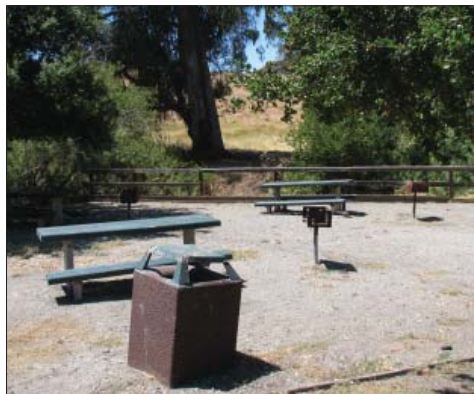
Picnic areas have become old and worn
