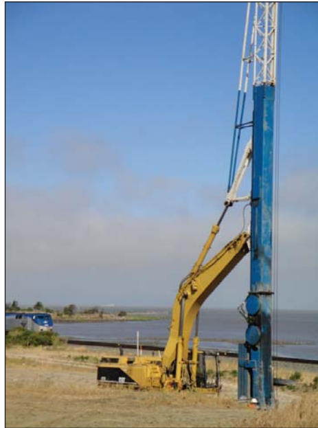
Special equipment is required for wicking, as seen here in Hercules
