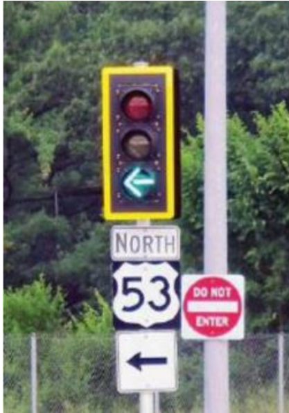
Figure 24: Retroreflective Backplates (Source: FHWA)
