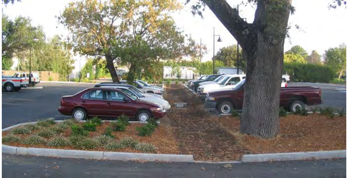
Photo of a bioswale used to treat and slow storm water runoff from a parking lot.
