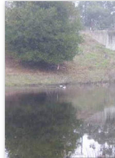
8. Detention basins on Hill Town site
