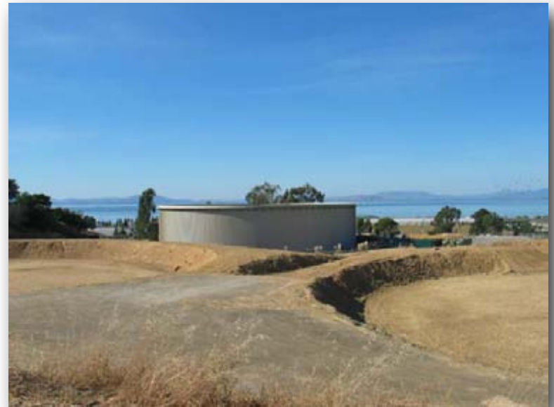
4. View west across Hill Town site with petroleum storage tank area
