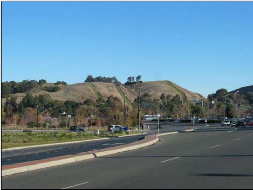
View northeast from San Pablo Avenue near Sycamore Avenue; Hill Town site in background
