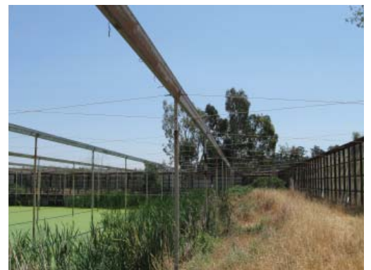
City's Corporation Yard in the Dynamite Project Area is ripe for redevelopment
